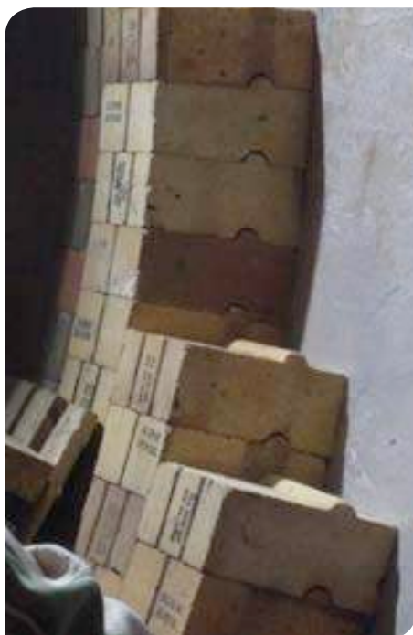
Below and Below Right - Figure 4: Lining of the tongue-and-groove bricks in the calcination zone.
