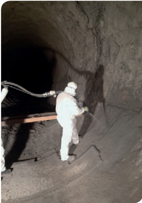
Right - Figure 3: Examples of veneering linings in the rotary kiln for cement clinker production.
