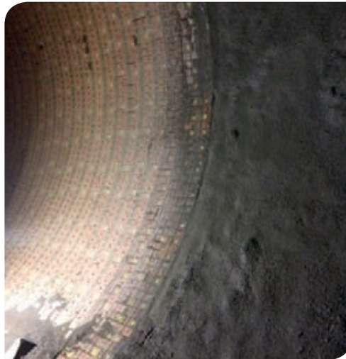
Right - Figure 3: Examples of veneering linings in the rotary kiln for cement clinker production.
