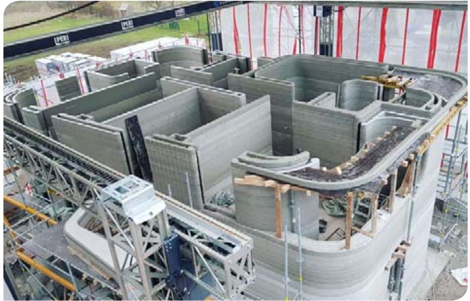
Above: Peri constructed the world's first three-storey 3D printed building in Germany using a BOD 2 Printer.
