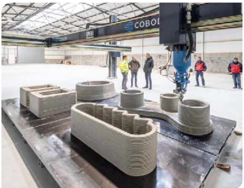
Below: 3D Printing opens up the possibilities of freeform building architectures.
