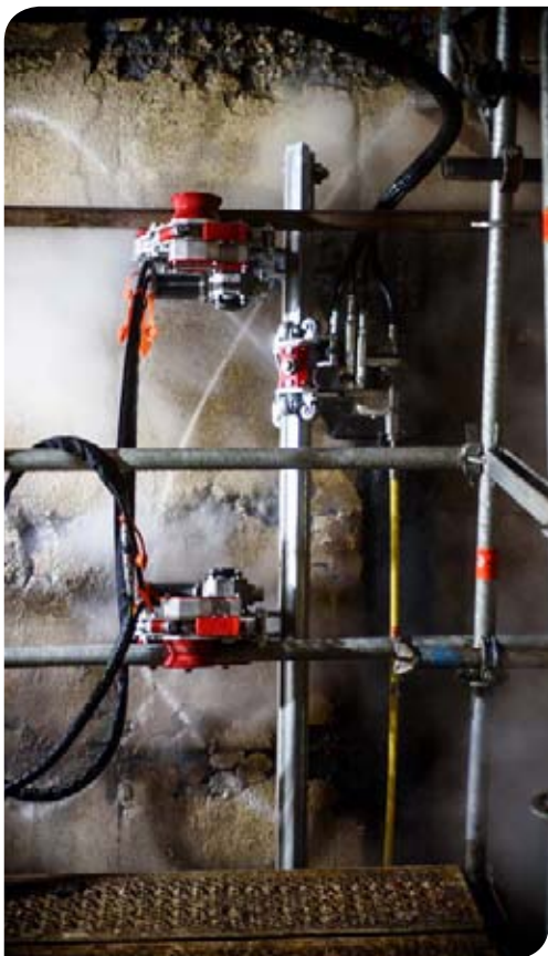
Above: Lightweight hydrodemolition systems are available that operate on a scaffolding system and provide four times the power of a hand lance.
