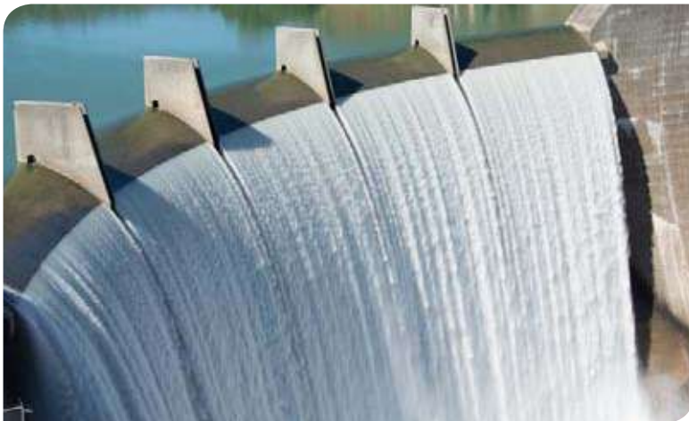
Above: Massive concrete structures such as dams require cements with low heat of hydration.
