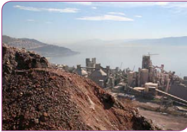
Above: The stunning view from the top of Nuh Çimento's marl and limestone quarry, looking over the plant and out to the Marmara Sea. The impressive plant is already capable of making 4.4Mt/yr of cement, with KHD's ball mill upgrade set to increase this further.
