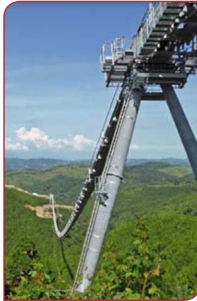
Above: The Dopplmayr RopeCon system was commissioned at Cementos Progreso's San Gabriel plant in April 2017.
