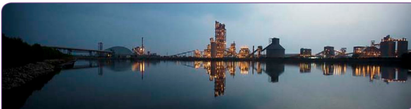
Below: The Orient Cement plant in Chittapur, Karnataka. Photo source: FLSmidth Pvt Ltd, entrant to the Global Cement Photography Competition.
