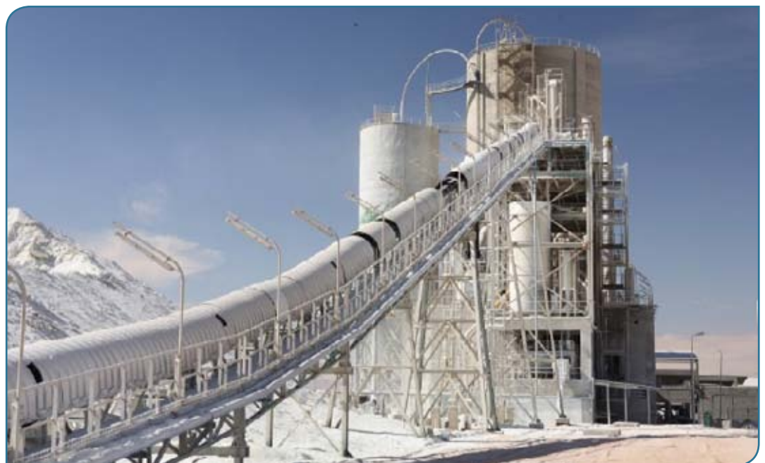
Below: The Sinai White Cement plant in Egypt. Many Egyptian cement producers have rushed to use coal in recent years following a curtailment of gas subsidies. Have corners been cut in terms of safety in the quest for speed?
