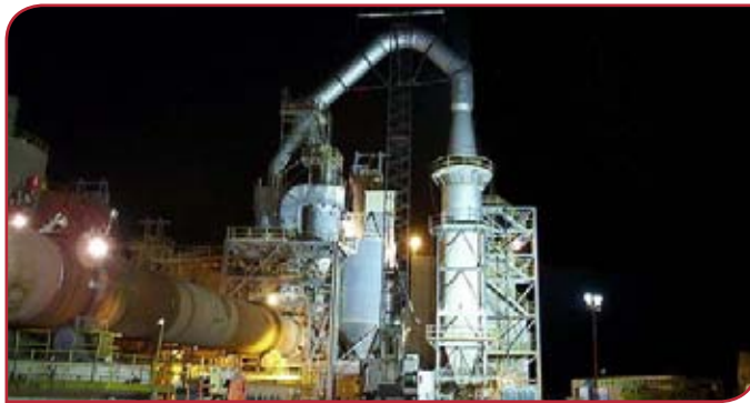
Above: Nevada Cement was fined US$500,000 for violating the Clean Air Act.
